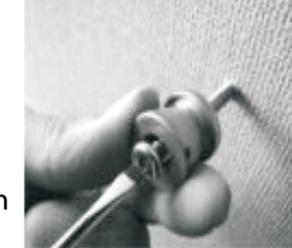
9. Insert the long screw (4) through a bush or short tube (3), then screw into the wall anchor (5).
