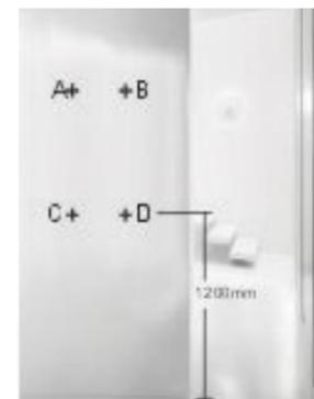
6. Mark the location of A, B, C, & D. It is recommended to install the towel warmer a minimum of 600mm from the floor.
