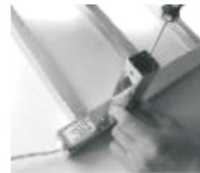
3. Screw down the short screw (6) with a screwdriver. Note that the hole of the bracket (1) should face towards the floor when the towel warmer is mounted.
